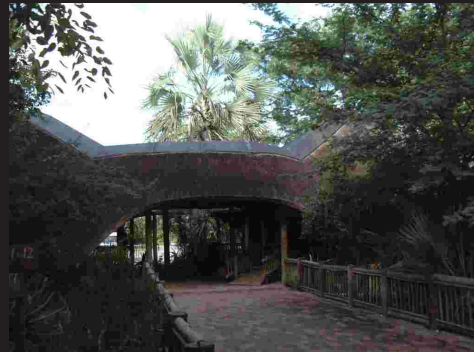
Approach to reception area from courtyard
